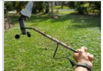
Data Marine Wind Vane Repair (Third time) 2013
