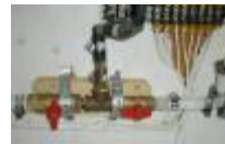
Fresh Water Flushing
