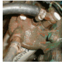
Bleeding the Fuel
