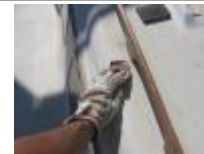
Painting the Deck Nov 2008
