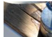
The Teak work has started Nov 2008
