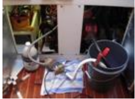
Heat Exchanger Cleaning-In Place
