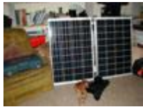
Installing Solar Panels
